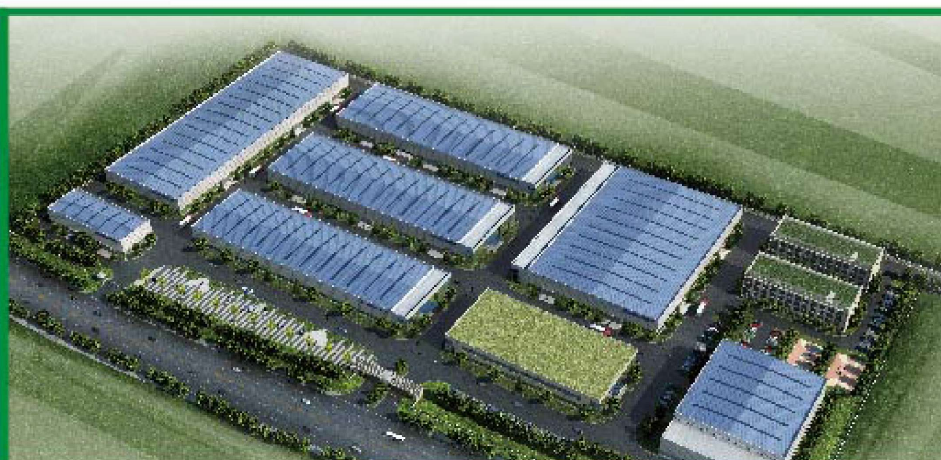
Hubei Factory (under construction)
